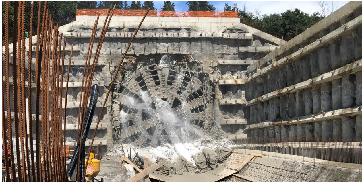
Image 9. Final break-through of the TBM
