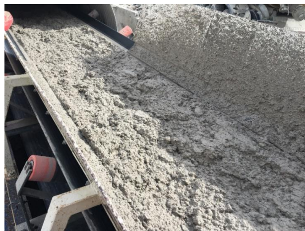
Image 7. TBM excavation through the “Sillano” geological formation.
