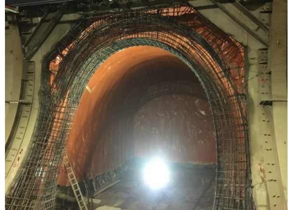
Images 2 and 3. Segment production with Dynamon NRG1015S and one of the niches waterproofed with Mapeplan TU20.
